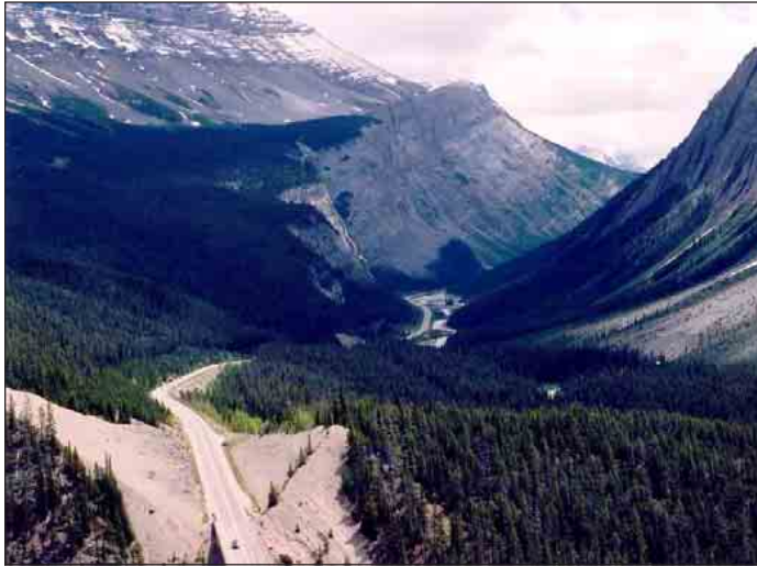
Highway 93, the Icefields Parkway, Alberta, Canada
